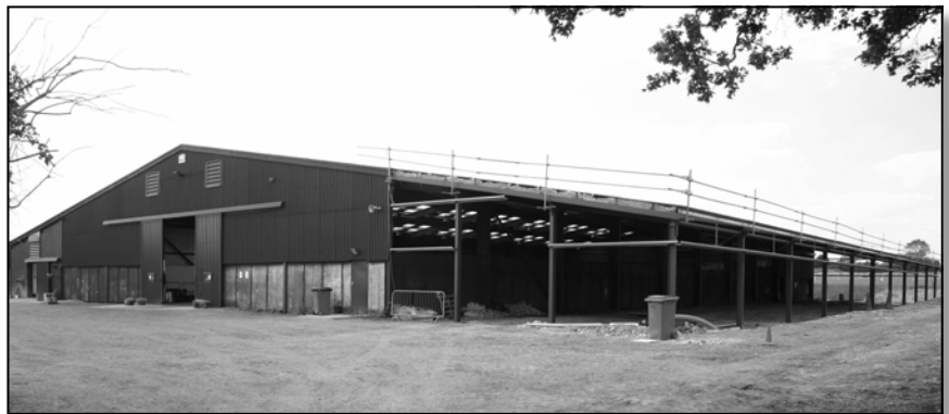
Work in progress to extend the facilities at NH
