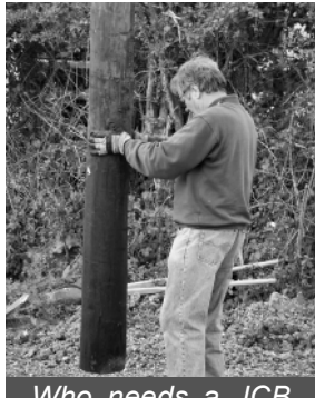
Who needs a JCB when Les easily lifts a telegraph pole into position on the lorry park
